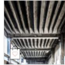
Rippenplatte Stahlbeton / L=6.84m, B=1.495m
