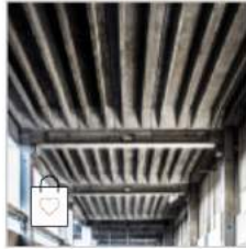
Rippenplatte Stahlbeton / L=5.79m, B=1.495m
