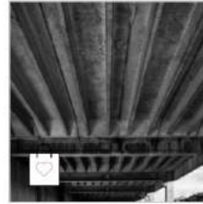
Rippenplatte Stahlbeton / L=5.99m, B=1.495m
