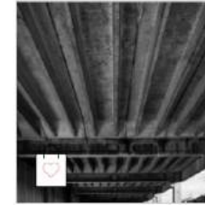
Rippenplatte Stahlbeton / L=8.97m, B=1.495m
